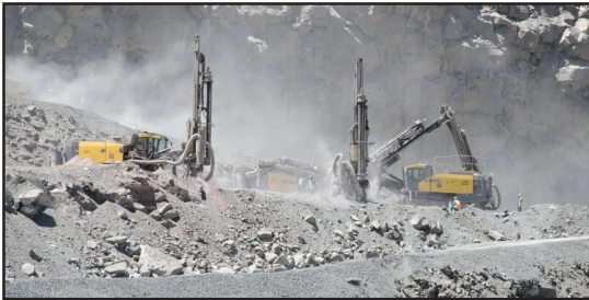
A mine where ACB units are installed.
